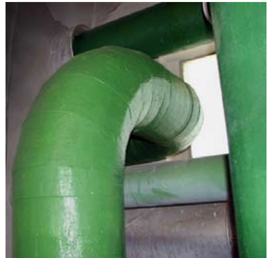
Aerogel insulation was thin enough to use on all bends in the piping and in the most confined areas. Green finish was easily applied to identify fluid inside.
