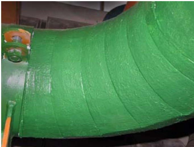
Aerogel insulation was thin enough to use on all bends in the piping and in the most confined areas. Green finish was easily applied to identify fluid inside.
